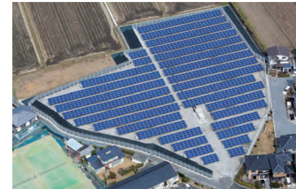
Higashi-Omi City, Shiga Prefecture / Flat site Solar cell capacity: 552kW
